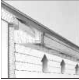
Figure 5.3 Undereave Soffit Vents
